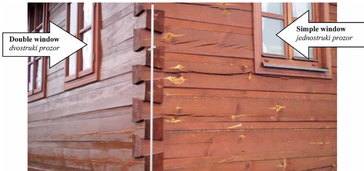
Figure 1 A view of simple and double windows from the exterior Slika 1. Pogled na jednostruki i dvostruki prozor s vanjske strane
